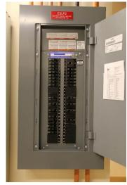
the small loads typically served, lighting and appliance panelboards will typically house a large quantity of singlepole overcurrent protective devices as compared to multipole overcurrent protective devices.
