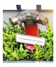
be located in a readily accessible and visible location to the fire department access of the building. The FDC is used by the fire department to connect fire hoses from a pumper truck to supplement the water supply to the fire sprinkler system in the building.
